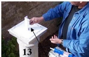
Tilting the column to one side may make it easier to position the rod so it can be inserted through the hole in the cap. Make sure that the attached angle is oriented properly. Caulk around the center hole. Only finger tighten the stainless steel nut at this time.
