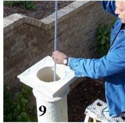
Lower the threaded rod into the column and engage the coupling nut on the bottom
