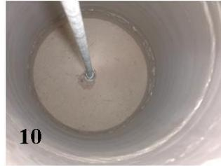
Screw the threaded rod snugly into the coupling nut at the bottom of the column and tighten with pliers.
