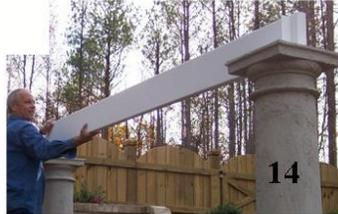
Install the headers **without** decorative rafter tails on the opposite side of the aluminum angle using the 2.5" hex head stainless steel screws. Set the clutch on the drill so the screw is not stripped.
