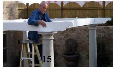
Install the headers **with** the decorative rafter tails on the opposite side of the aluminum angle using the 2.5" hex head stainless steel self tapping screws. Set the clutch on the drill so the screw is not stripped.
