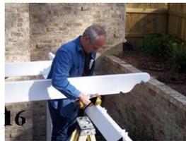
Starting in the center of the arbor begin installing the rafters with the decorative tails. The headers have fiberglass angles as shown which indicate the rafter location.
